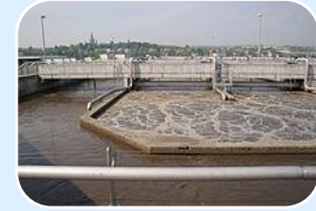
Waste Water Disinfection
